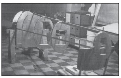
A second D–8 fuselage being built in Glenn's basement confirmed to Lloyd that the construction and jigging requirements were straightforward enough for cadet builders.
