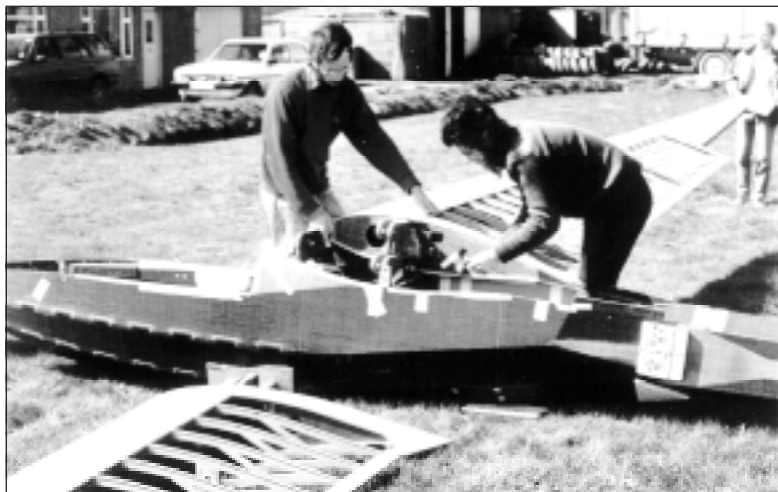
Early rigging tests on the partly assembled prototype. Tabs along the fuselage panels that create the interlocking, self-jigging joints are evident.
